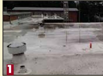
Replace and/or repair flat roofs on courtyard, rectory, and school to allow for correct drainage and eliminate future leaks.
